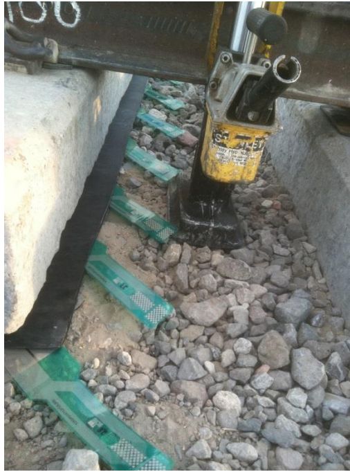
Figure 7.5 Pressure sensors being installed under raised track
